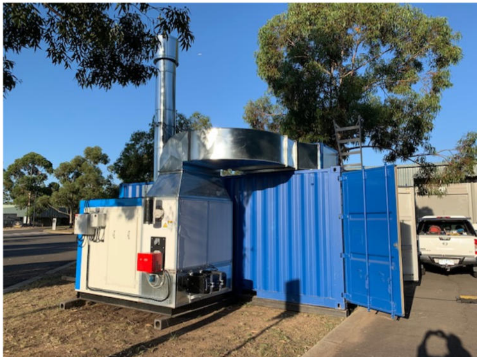
HEATING POD UNIT - DIESEL FIRED HEATING 25.C WITH OPTIONAL 40.C BAKE
