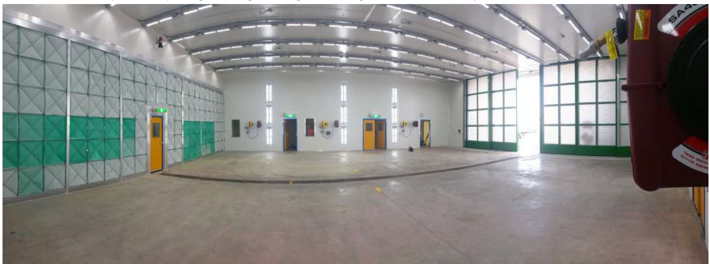
Above: Internal viewpoint of facility showing wide expanse of space & lighting to provide operators with a safe and compliant space.
