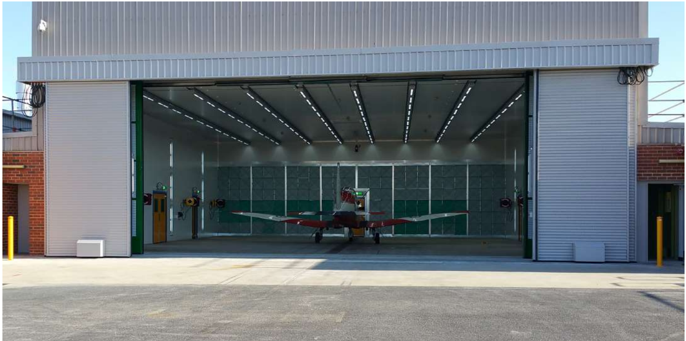
Above: External viewpoint of the painting cabin, large dual stage doors integrated into booth & facility.
