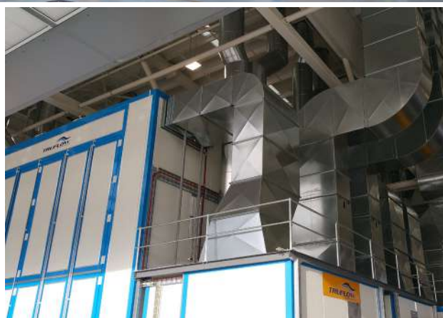
Above: Multiple views of the large scale downdraft facility showing the booth, mechanical ductwork, service platforms and internals.
